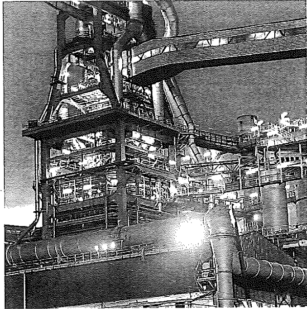
Industrial application: Refinery
